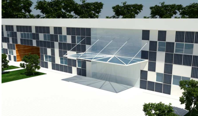
Fig. 9. Photovoltaic panels generating electric power located on the southern facades of the building
